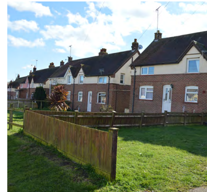
Figure 39 Twentieth century semi-detached houses
