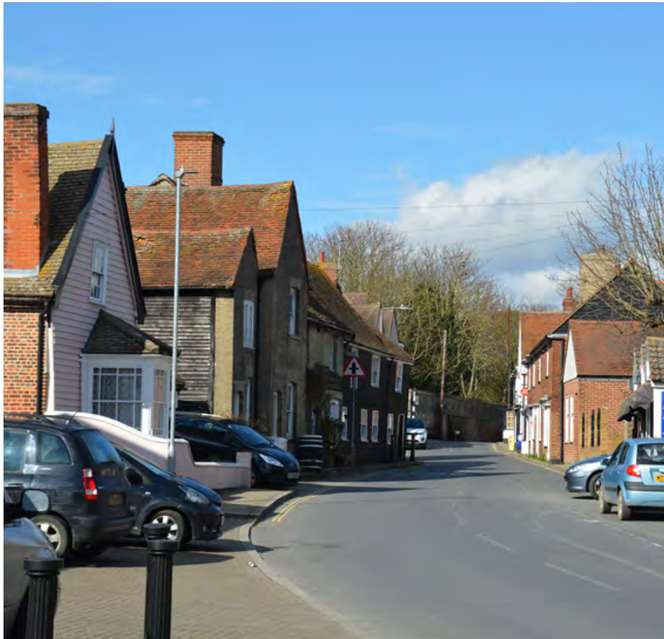
Figure 43 View towards Bar Corner
